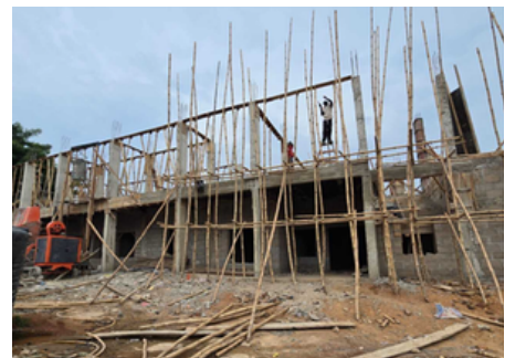
Main CTU under construction at AEFUTHA, Abakaliki, Nigeria
